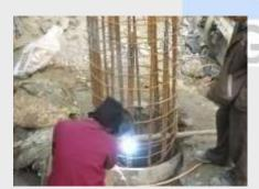
Under reamed piles – this pile is basically developed for black cotton soil and used for light structures.
